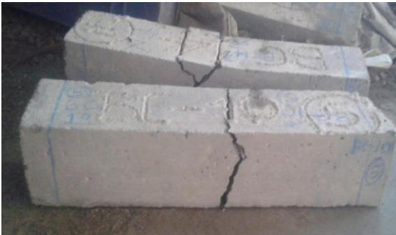
Failure pattern of reinforced concrete beams
