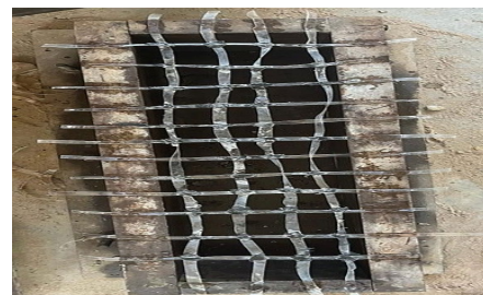
Fig.3. Preparation of plastic reinforcement
