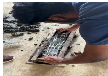
Fig.4. Placing of plastic reinforcement
