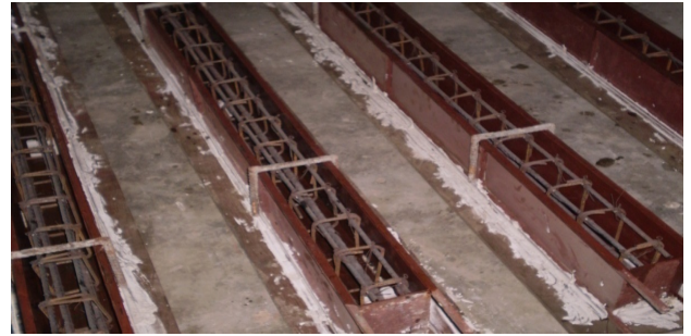
Fig 4.3: Beams ready for concreting
