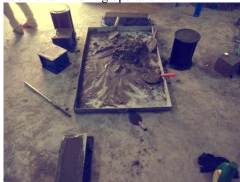
Fig 3.13 Finishing of concrete
