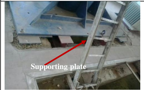
Figure (2-a) Stiffeners and Supporting Plates
