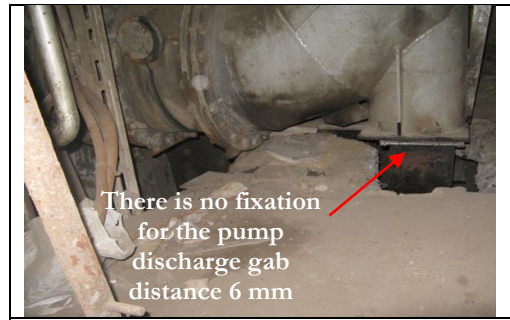
(a) There is no fixation for the pump discharge gab distance 6 mm
