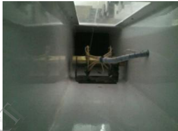
Figure 3: Fin assembly inside the duct
