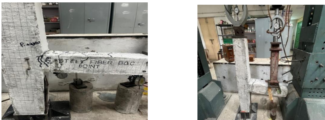
Fig. 9.1.2 Cack patten and Failure modes of Steel Fibre Beam and Column Joint
