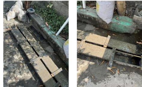
Fig. 9: Placement of internal steel reinforcement cages inside the beam molds with proper concrete cover
