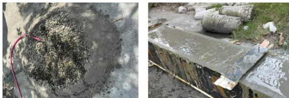
Fig. 8: Materials for the concrete mix design used for all beam specimens
