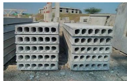
Fig. 2. Hollowcore Slab System
