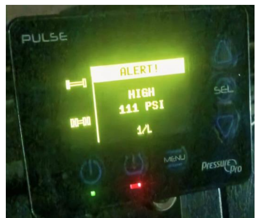
Fig-8: Display Unit at Operator Cabin
