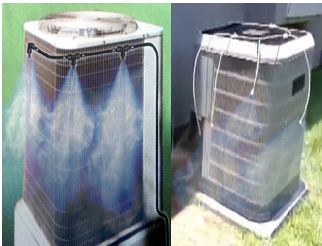
Figure3. Adiabatically pre cooling using condensate water
