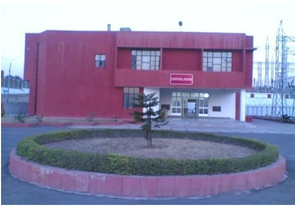
Fig. 2 Control room of Barn Grid Station
