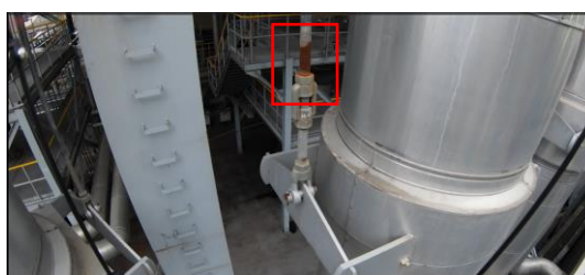
Figure 14. Minor corrosion on hanger rod.
