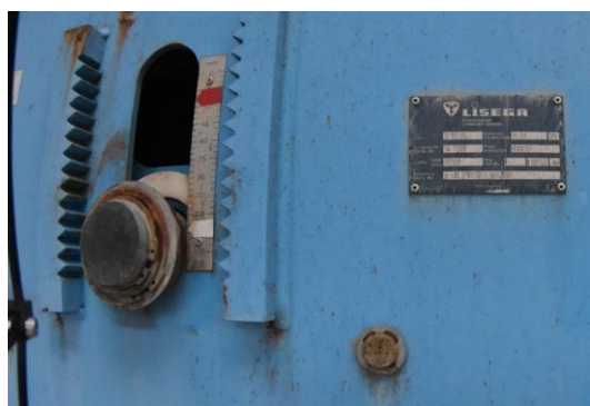
Figure 9. Alost bottom over-scaled hanger travel and visible hanger nameplate.
