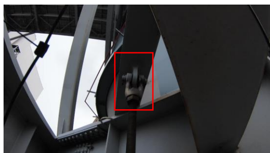
Figure 12. Condition of hanger clevis, lock nut, clevis bracket.
