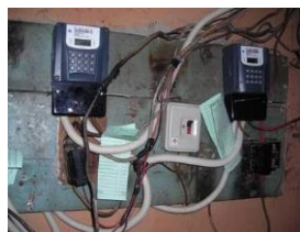
Figure 3.b. Tampering with the meter
