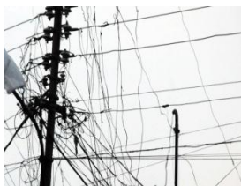
Figure 3.a. Hooking/Tapping
