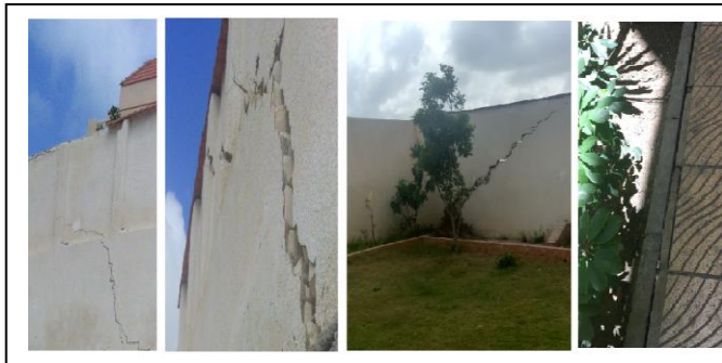
a. Test C near longstanding construction strip foundation
