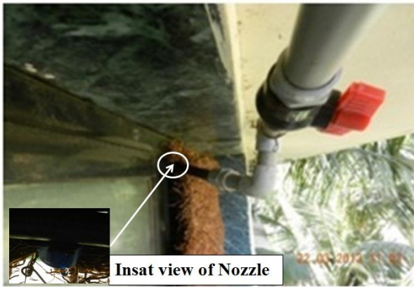
Fig.3 Water dripping arrangement
