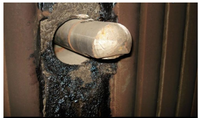
Fig.3: view of soot blower inside furnace
