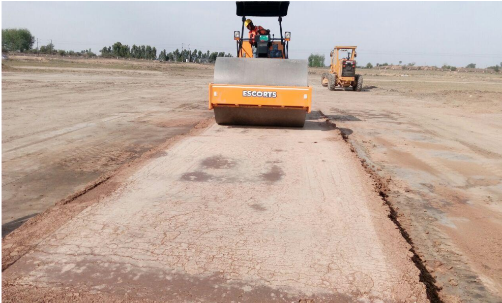
Compaction of Trail Bed Vibratory Roller Figure No.3
