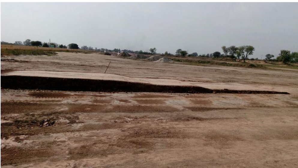
Prepared Trail Bed of Varying Thicknesses of 150mm, 300mm & 450mm Figure No.4
