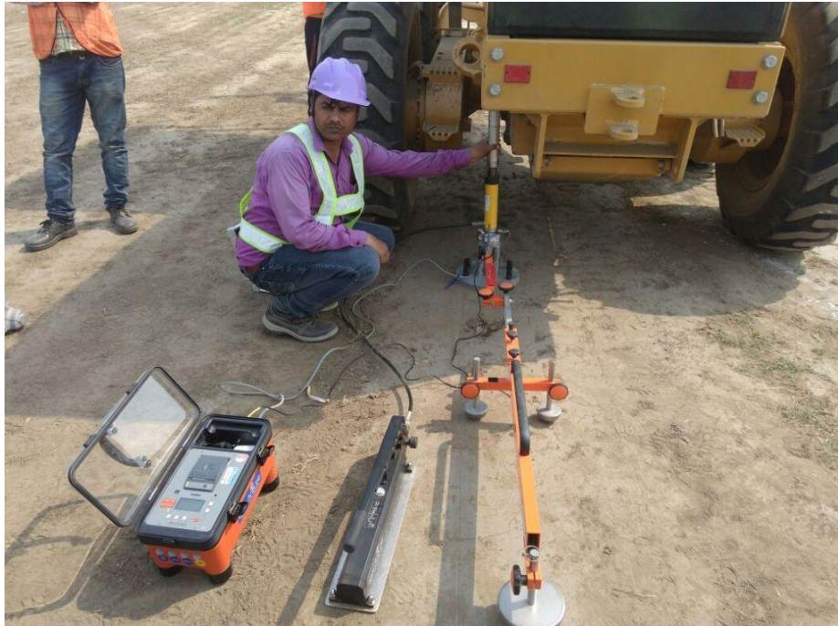
Field Testing of Strain Modulus (EV2) on Natural Ground. Figure No.5
