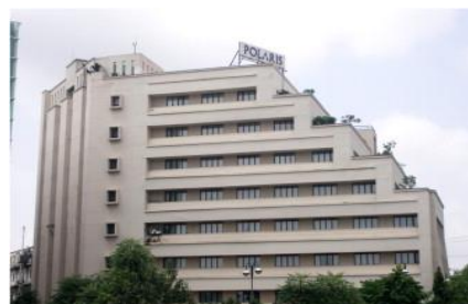
Fig.1. Stepped building frame
