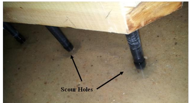
Fig. 9. Scour holes around piles
