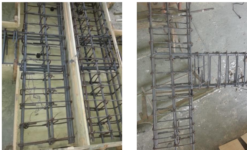
Figure (4): Reinforcement cages, formworks of joints.
