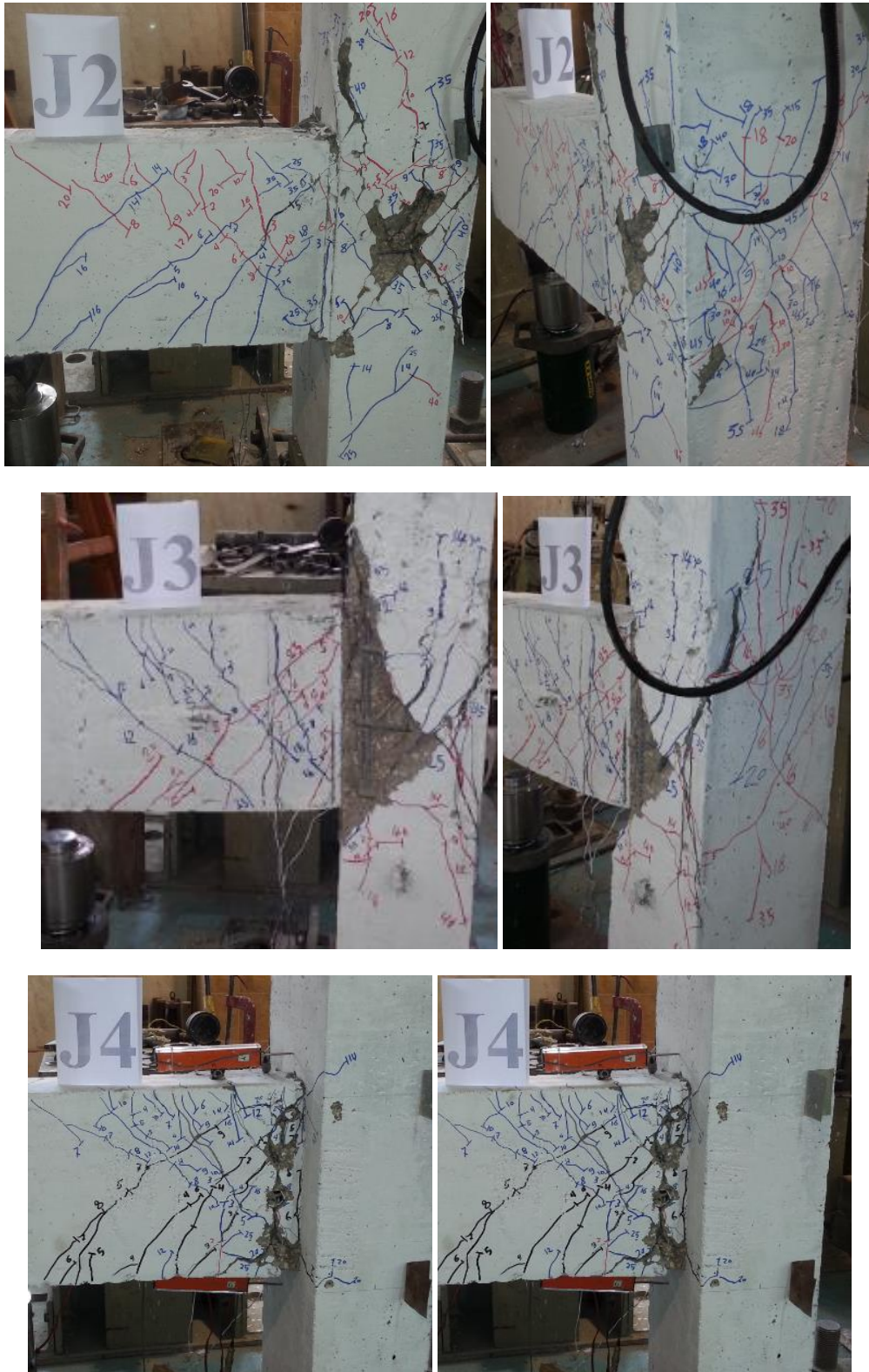
Figure. (8) Cracks patterns and failure mode of joint (J2, J3 and J4).
