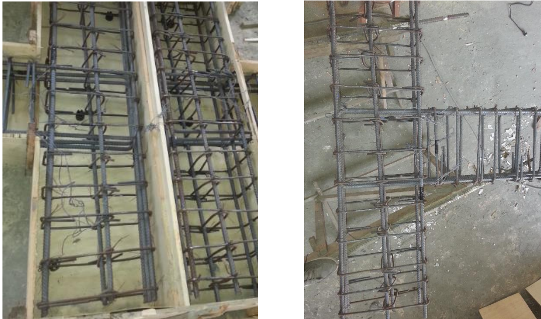
Figure (4): Reinforcement cages, formworks of joints.
