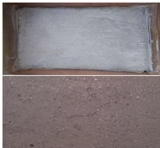
Fig: 8 Crack assessment of shrinkage slabs
