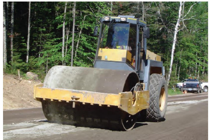
Fig. 1 – Rolling of Cement Treated Granular Layer
