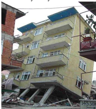
Fig2.a:Soft storey effect in Düzce1999[2]
