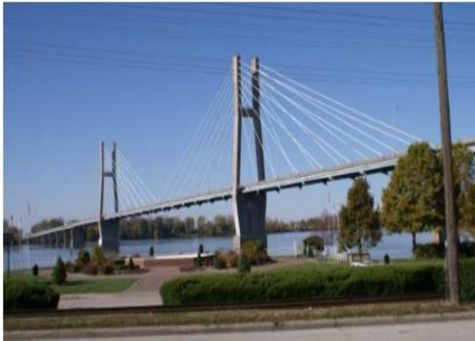
Figure 5: Quincy Bayview Bridge
