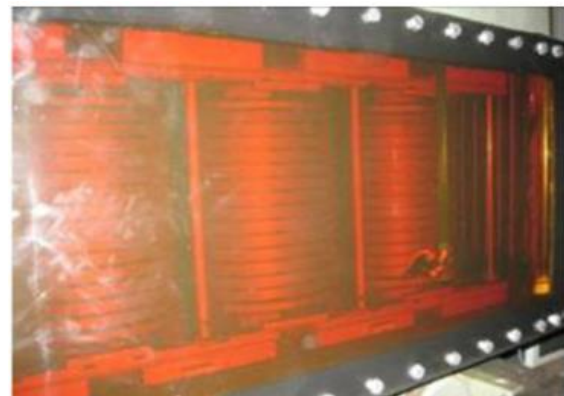
(b) After refilling the oil to the tank.
