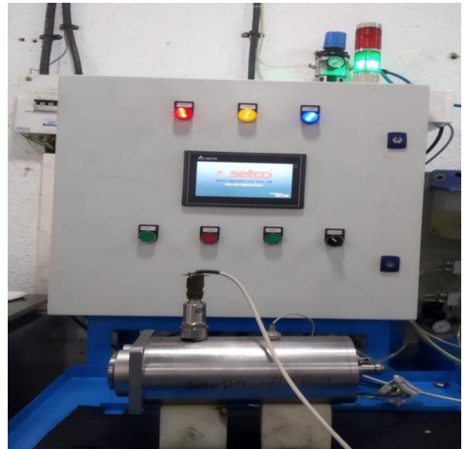
Fig.3 - Front view of PLC based Automated Spindle Testing Platform
