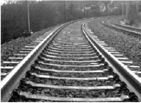
Figure 7.2: Carbide-free bainitic steel in service. Swiss Railways using new rails [11].
