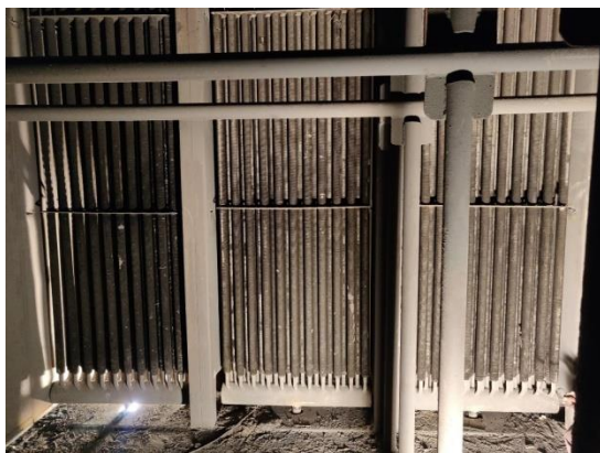
Figure 19: SCAPH post modification in closed position at site (causing pressure drop)
