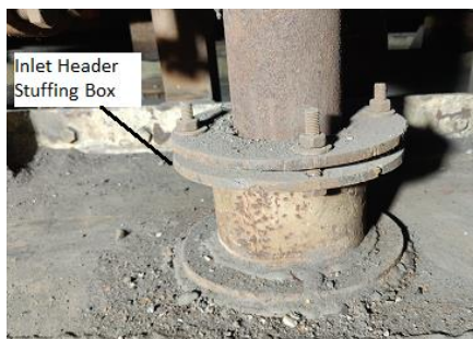
Figure 11: Inlet Header Stuffing Box
