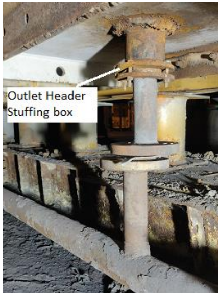
Figure 10: Outlet Header Stuffing Box
