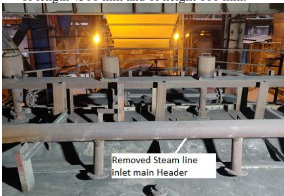
Figure 7: Steam Line Header
