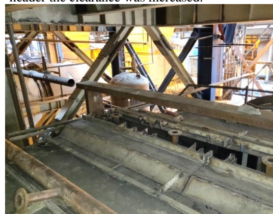
Figure 9: Modification of forced draft fan outlet duct
