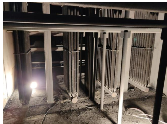
Figure 20: SCAPH post modification in open position at site (causing no pressure drop)
