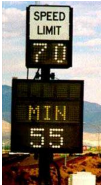
Fig. 4: Variable speed limit sign
