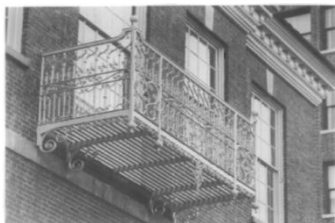
Figure(4). Wrought-iron Balcony, Samuel Wheeler, blacksmith; Congress Hall, 1787-1789..
