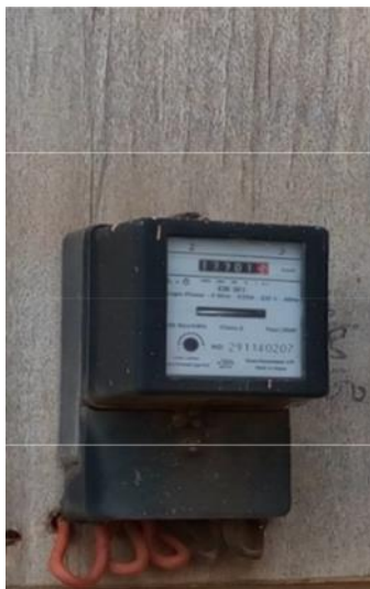
Fig. 2. Electromechanical Energy Meter
