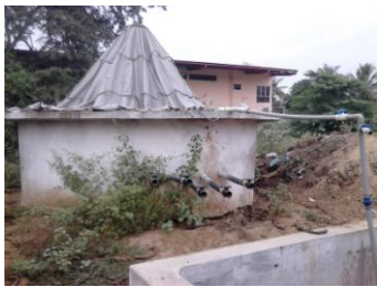
Fig. 3 Balloon type biogas plant
