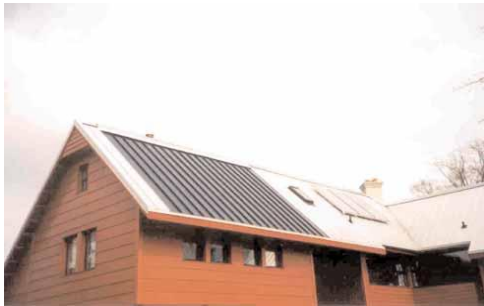
Fig.17 BIPV metal-standing seam roof, Toronto
