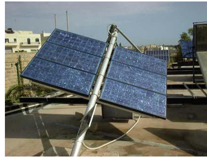
Fig.15, A 360 Wp single-axis PV tracking
