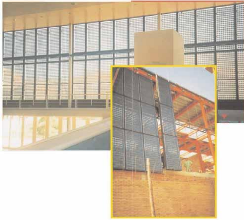
Fig.16 PV integrated in curtain wall elements at the Mataró Library, Mataró, Catalonia, Spain. (The facade is also used for fresh air pre-heating).
