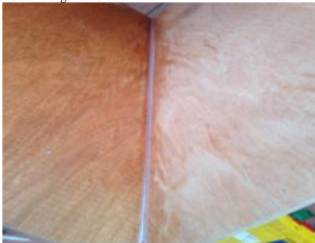
Fig. 27. Filling of gaps using Silicone Glue
