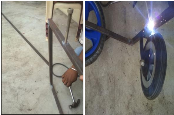
Fig. 3. Photos captured during fabrication of sprayer frame
