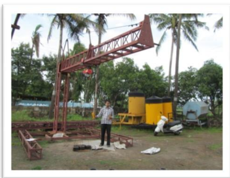
Fig. 3.3 Testing of Crane
