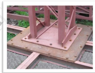
Fig 1.5 Design of column bases with bolts
