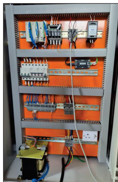
Fig. 6. Control panel wiring and PLC integration
