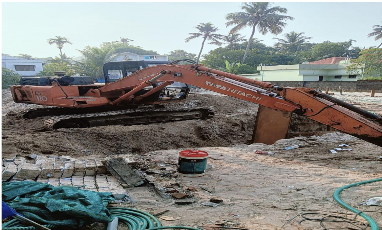
Fig 1.7: Commercial building for Mr. Faby Varghese at Cherthala
