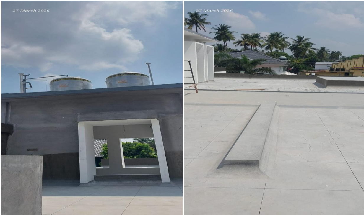
Fig 1.6: Residential building for Mr. Rinto Moyalan at Ollur
