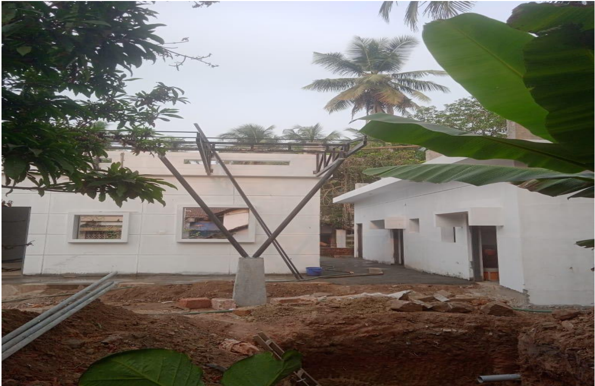
Fig 1.10: Construction of LP School at Vellayil, Kozhikode
