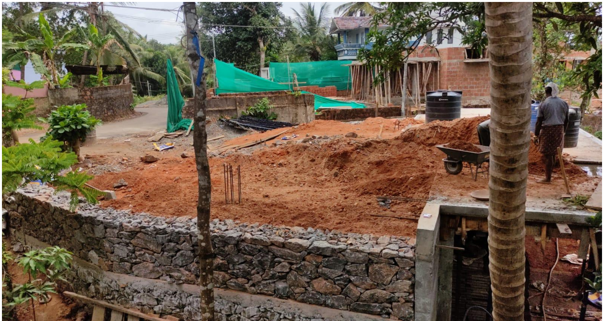
Fig 1.9: Construction of Subcenter at Melangady, Malappuram by HLL
