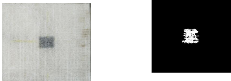
Fig.10. Delamination at center, a) Original image, b) Processed Image
