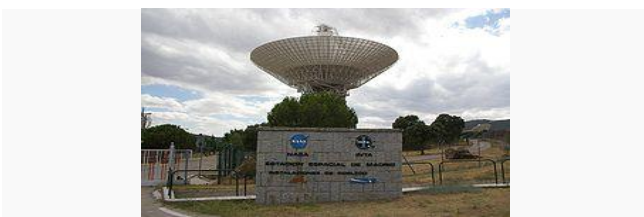
Fig 3: 70m antenna in Robledo de Chavela, Community of Madrid, Spain
