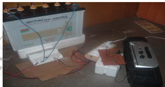
Fig 8: Trial with 12V,75AH battery
