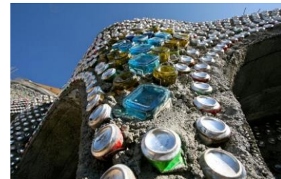
Fig. 3. Using Aluminium Tin Cans for wall construction
