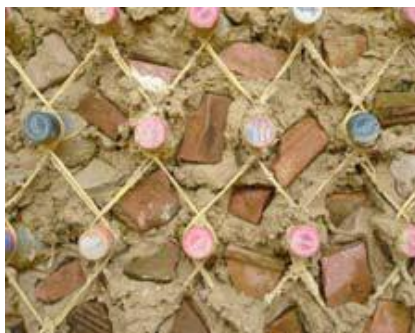
Fig. 6. Plastic bottles tied with nylon rope and binded with construction waste and other local binders (Eco-technologie, projects, 2014)
