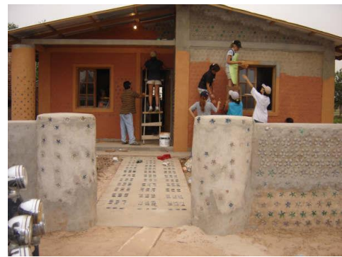
Fig. 1. Construction with PET bottles, Honduras
