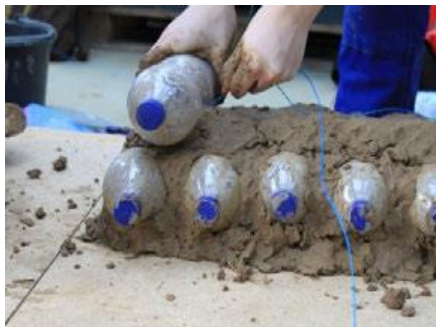
Fig. 5. Plastic bottles being laid for wall construction (Volker et al., 2012)
