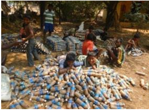
Fig. 4. Plastic bottles filled with dry soil (Samarpan foundation, 2021)
