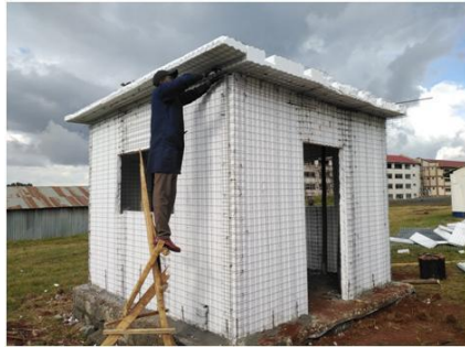
Fig. 1. Walling of model house using EPS Panels
