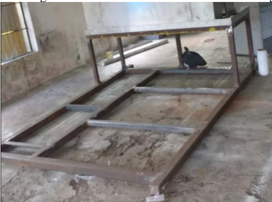
Figure no. 12. Fabrication of Base and Support
