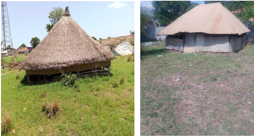
Figure 1.1 A typically examples of Huts sinks in black cotton soil in Bor
