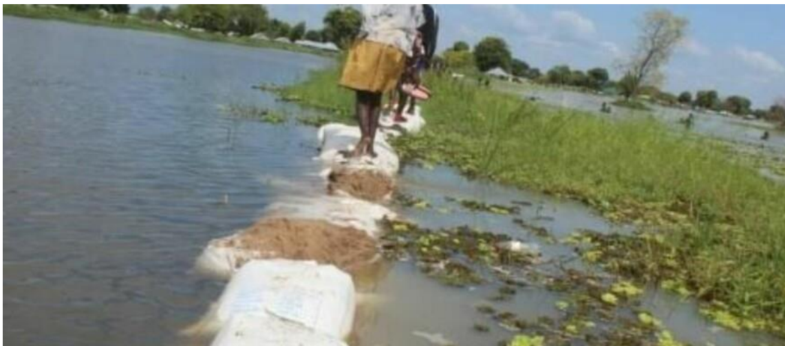
Fig 5.1 A dyke that was overtaken by Nile River waters in Bor. Waterlogged: Flooding reduced bearing capacity of black cotton soils. When dry, its strong but lose their strength when saturated. Waterlogging can weaken the soil's bearing capacity and increase the risk of foundation failure making them unsuitable for supporting structures, especially in flood zones. Soil Swelling: Black cotton soil is acknowledged for its expansive nature. When it absorbs water during flooding, it tends to swell, increasing in volume. This Impact on Buildings leading to ground heave and settlement, causing structural damage, cracking in walls and foundations, and even potential collapse in many cases. Increased Saturation: Flooding causes the soil to become saturated, leading to an increased risk of hydraulic conductivity issues, the drainage becomes very slow. Saturated soil can lead to shallow foundations instability due to hydrostatic pressure on foundation walls can also increase, potentially leading to structural failure. Erosion soil: Floodwater can cause soil erosion, especially on slopes or near stream beds. This impact on Buildings, leading to settling or tilting of buildings. Over time, erosion can significantly challenge the structural integrity of buildings. Drainage Issues: Black cotton soil has poor drainage properties, meaning it retains water for longer periods. Poor drainage aggravates the effects of flooding, increasing the duration of water sitting around or under the structure, leading to prolonged periods of risk for flooding-related damage.
