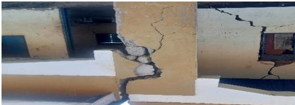
Fig 1.7 Typical black cotton soils structural damage, school buildings in Bor Town Road Pavements and Damage: the swelling and shrinking of black cotton soil can cause potholes, cracks, and other damage to roads and pavements. Due to very low CBR values of black cotton soil, excessive pavement thickness is required for designing for flexible pavement. The constant stress and strain from loaded transport vehicles are most liable to damage as a result of the volume changes in the soil. Dampness: moisture issues it's crucial causes building materials to deterioration, corrode, and weaken, reducing their lifespan. General Site Descriptions: The Studied Area is located in the capital city of Jonglei State, Bor Town, where area lies is seen as extensive plain clay that is associated with the White Nile. The area is part of the semi- arid climate, which is hot and dry with summer rain and a cold dry winter season. The study area is composed mainly of superficial clay deposits and alluvium of the White Nile the clay mineralogy of the study area is strongly dominated by Smectitic clay minerals mainly montmorillonite type, which is an expanding clay mineral. Topography: The land form of the study area is almost flat and hence flooding usually stances for a lengthy time after rainfall. Therefore, surface drainage is necessary to be considered. The major kind of land use includes rain fed agriculture such as traditional and mechanized farms of sorghum and irrigated agriculture such as fruits and vegetables. White Nile River and its flood plain and rain water constitute the main sources of flooding in the area, since the study area lies on the western bank of the White Nile. Drainage Patterns: Black cotton soils in Bor, Jonglei, and some areas of South Sudan in general, exhibit impeded drainage due to their high clay content and low permeability. This makes them prone to waterlogging and can hinder the construction of buildings and other infrastructure. The poor drainage of black cotton soils can lead to waterlogging, which can affect the growth of crops and cause issues with sanitation, hygiene, and pose significant challenges for construction, making it difficult to build stable foundations and infrastructures.
