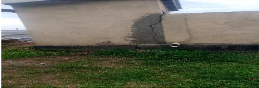
Figure 1.6 depicts a washroom at Greenbelt Academy in Bor Town. Structural Damage: The ongoing cycle of expansion and contraction can result in visible cracks appearing in the walls, floors, and ceilings of structures. Over time, this deterioration can jeopardize the building's structural integrity, potentially necessitating extensive repairs or, in some cases, complete demolition and reconstruction.
