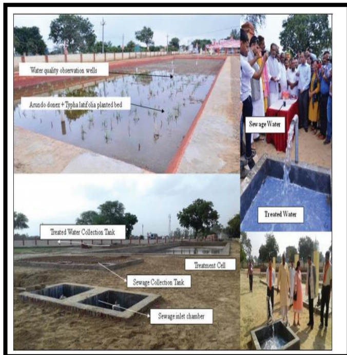
(Figure 9: Layout of Pilot Rural Household Sewage Water Treatment System)
