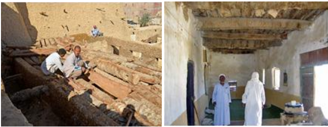
Fig. 3. Roof and interior restoration. [2]
