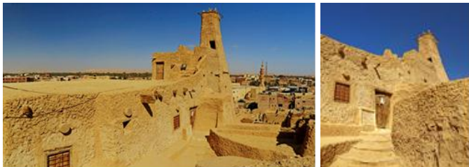
Fig. 2. Facades restoration using Karshif and Tafla finishing. Photographed by the researcher
