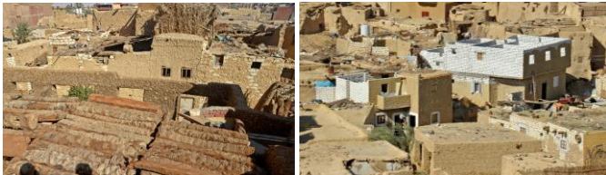
Fig. 8. New materials within old fabric, and New materials with mud finishing in Siwa, photographed by the researcher
