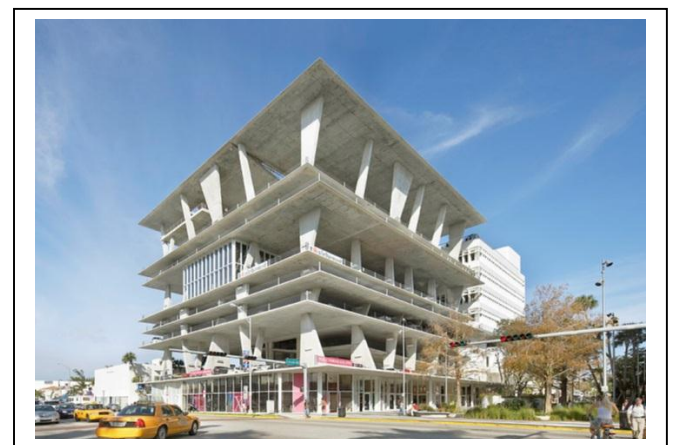
Fig. 4. Differences of height level floor of 1111 Lincoln Road [8]
