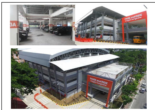
Fig. 3. The condition of Park & Ride building on Meyjend Sungkono Street. (suarasurabaya.net, 2017)
